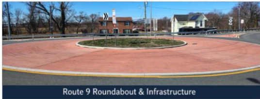
Route 9 Roundabout & Infrastructure
