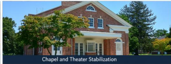
Chapel and Theater Stabilization
