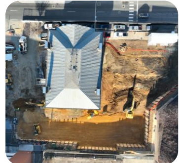
Brownfield Remediation, Fill, Compaction - 2025
